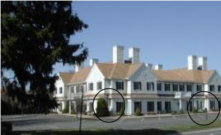
9300 square foot office condominium in Madison, CT uses gas-light style light poles
