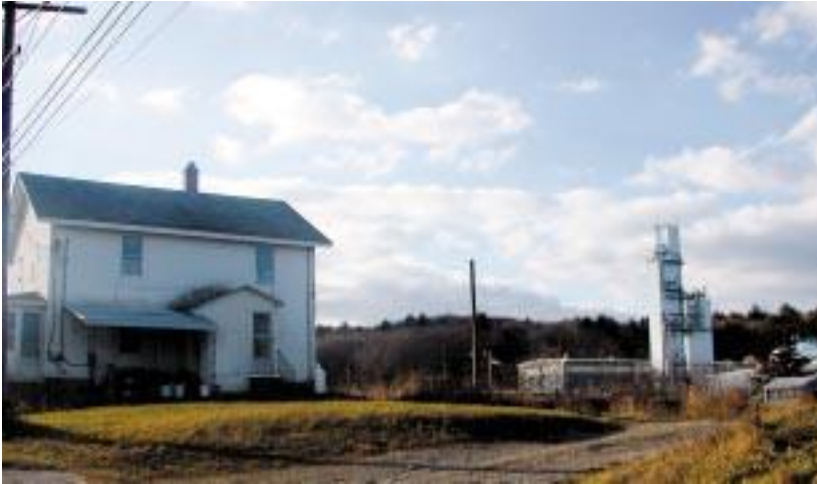
One- and two-story goat farm structures surrounded by AGA gas separation plant with five-story process tower, Bozrah, CT.
