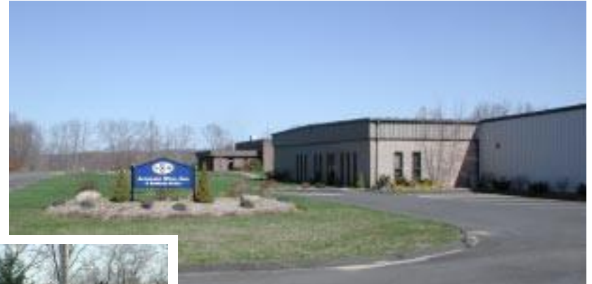
Industrial Park in Madison, CT: foreground building integrates stone front office with factory roofline by trim; background office building uses stepped slab and glass design.
