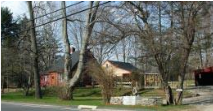
The professional office outbuilding follows the lines and uses the same materials as the home, Haddam, CT.
