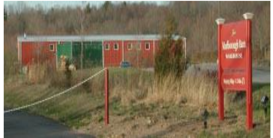
Tiny windows at the top of Marlborough Barn's warehouse office only emphasizes the unrelieved mass of the large building.
