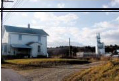
Goat farm and AGA Gas Separation Plant
