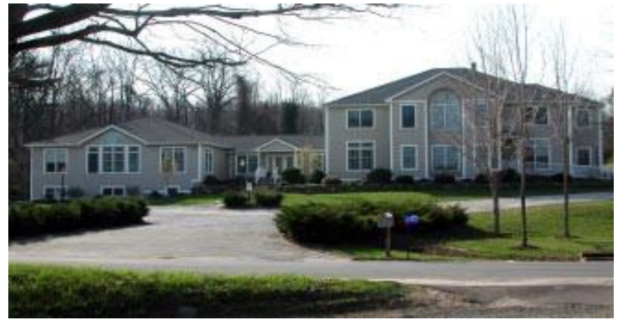
Marin Environmental Services, Haddam, CT is an excellent example of integrated multiple roof design
