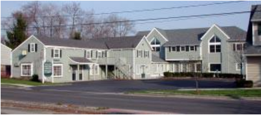
The larger professional office addition copies features of the pre-existing retail structure, Madison, CT.
