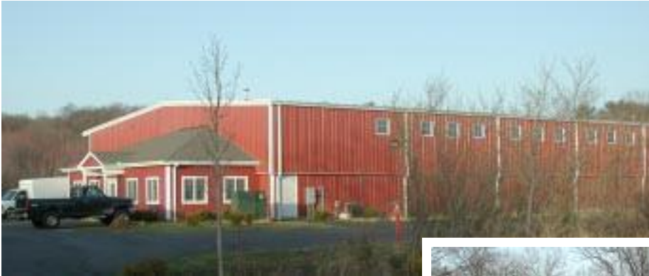
One-story office addition on the Marlborough Barn's new warehouse only emphasizes the unattractive mass of the larger building.
