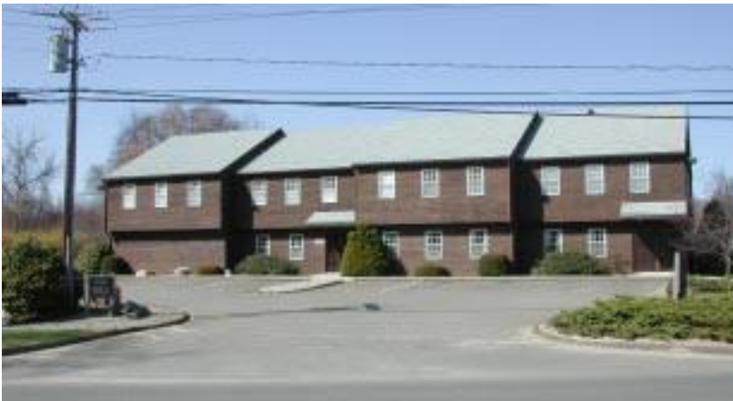
East Shore Medical Center in Madison, CT looks like a wall of boxes with no clear opening or entrance.
