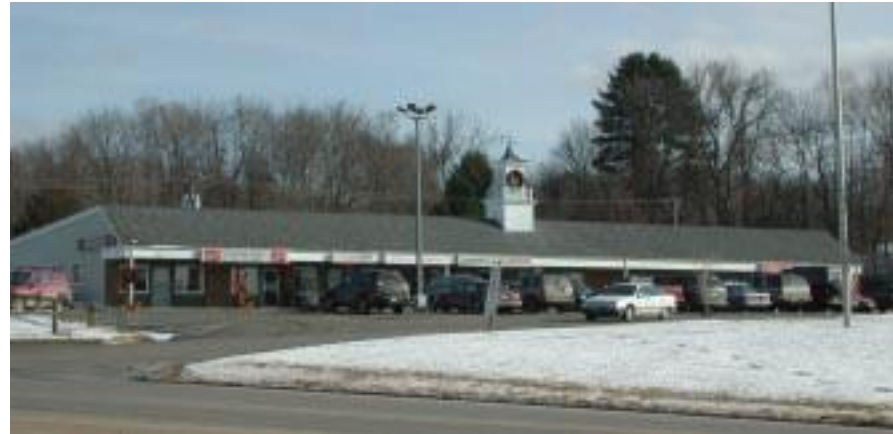
This strip mall in Moodus, CT has no building-related landscaping.
