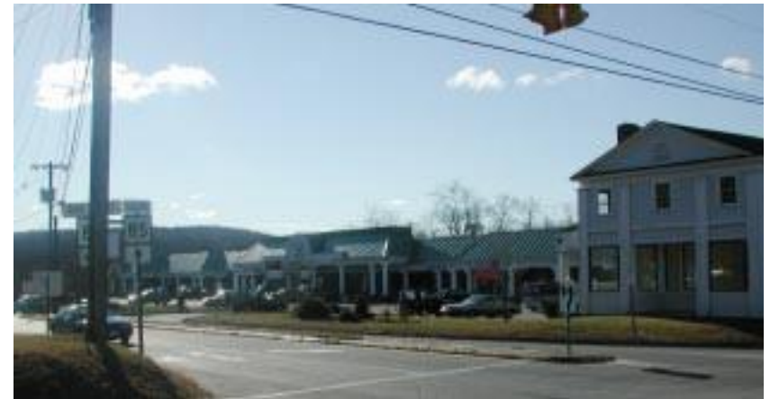
This strip mall at Salem Four Corners completely ignores the two-story historic commercial structure it surrounds.
