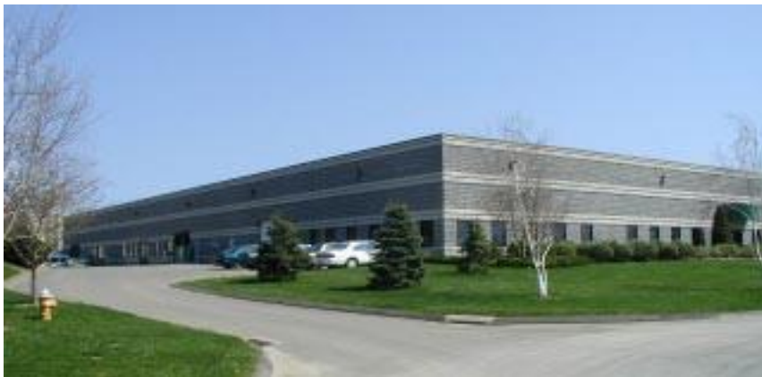
When mature, the evergreen and deciduous plantings will somewhat soften the visual impact of this 40,000 square foot, three-story industrial building in Old Saybrook, CT
