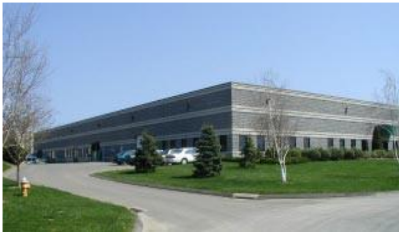
40,000 square foot multi-story industrial building, Old Saybrook, CT.
